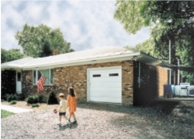
In July 1998, a single-family home in Latham, N.Y., was disconnected from its local electric utility and powered up with Plug Power’s 7 kW residential PEM fuel cell — the first house ever to do so. In August 1999, the system was converted to use the home’s incoming natural gas line as the fuel supply.
