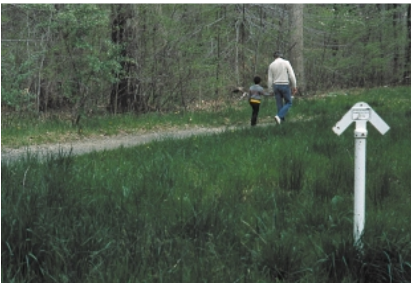
Underground natural gas lines leave little mark on the surrounding environment.
